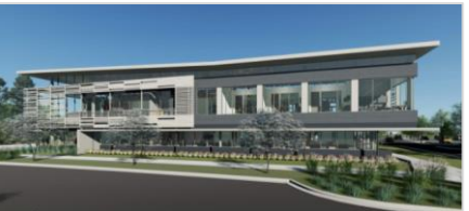
Florida Public Utilities Office
